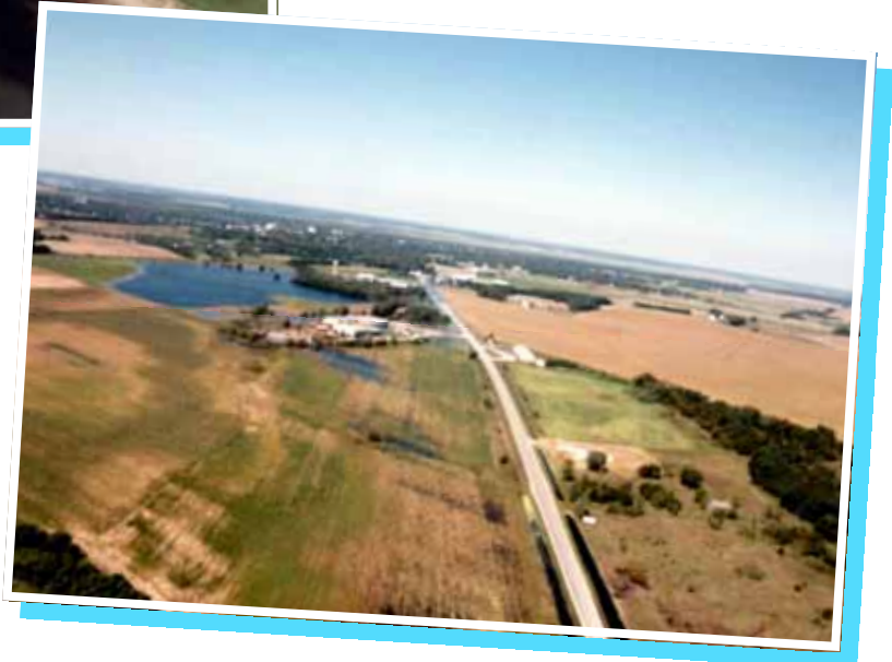
Looking north along IL Rte. 97 south of Havana
