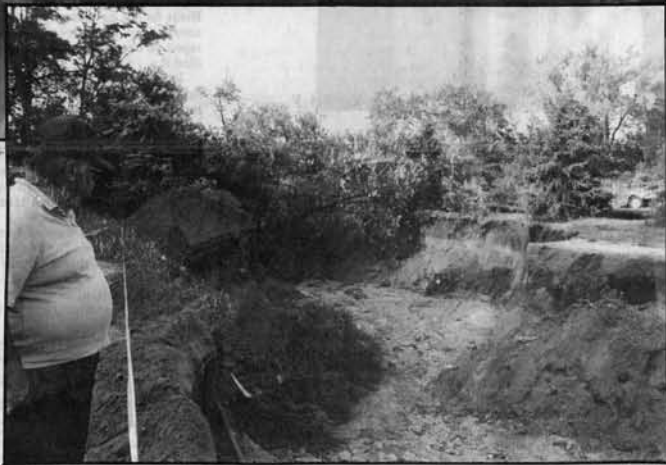
A gully washed out the end of Chestnut Street in Bath from the force of water flowing from a ditch that was dug to connect floodwaters in the village with the Bath Chute.
