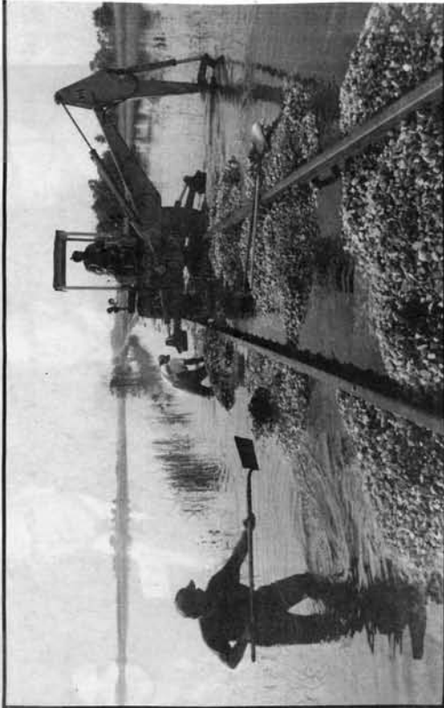
C&M Railroad employees used a special trenching bucket to scoop gravel from between railroad ties Saturday so that pipes could be placed under the track to aid in moving water out of the pond behind Walker Forge. Gravel had to be dug out by hand between the rails because high water prevented the trencher from reaching at the best angle.
