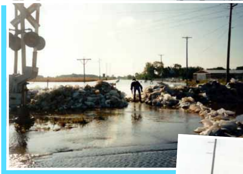
Looking south along IL Rte. 97 at the railroad tracks(southeast of Havana)
