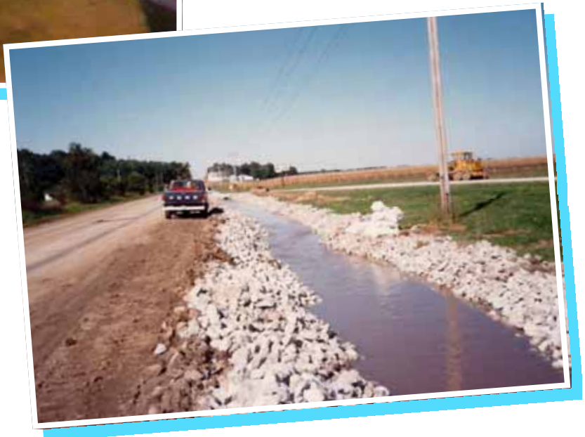
Finished drainage system in front of drive-in along IL Rte. 78
