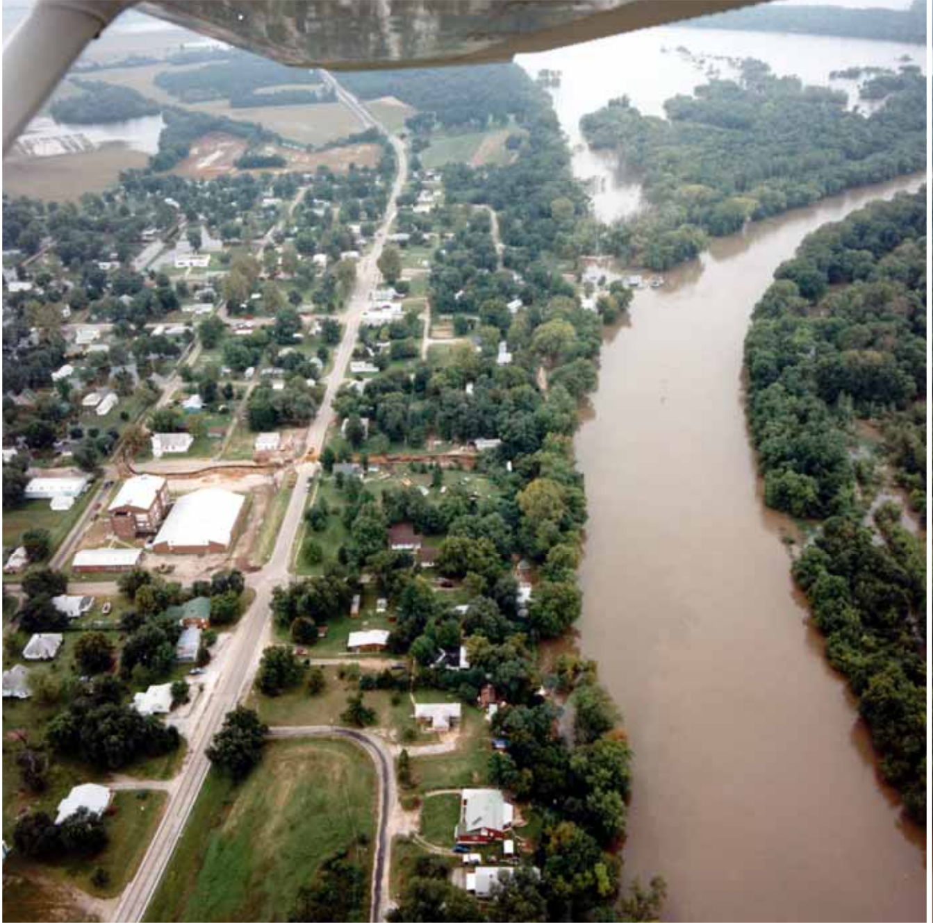
Looking south along IL Route 78 at Bath
