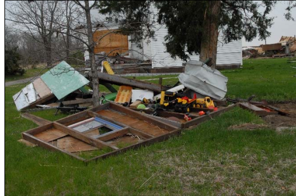
On April 15, 2011 an EF1 tornado near Poplar City destroyed several outbuildings, including this garage.
