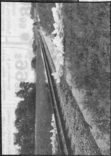
Sand bags at the C&M railroad were used to keep south and east ends of water from running down Havana.
