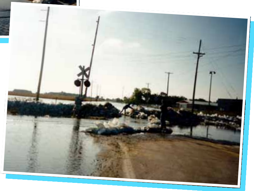
Looking south along IL Rte. 97 at the railroad tracks (southeast of Havana)
